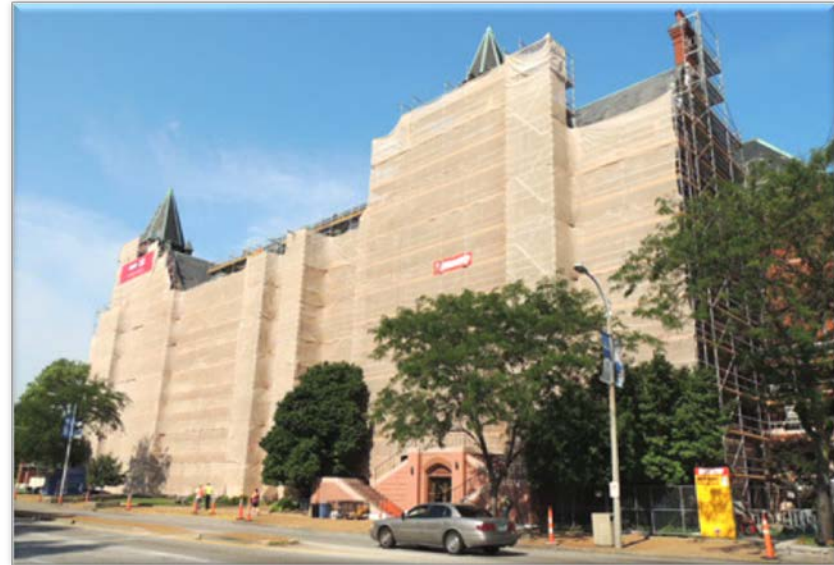
Covered scaffolding surrounding DuBourg Hall during masonry and tuck-pointing repairs in 2014.
